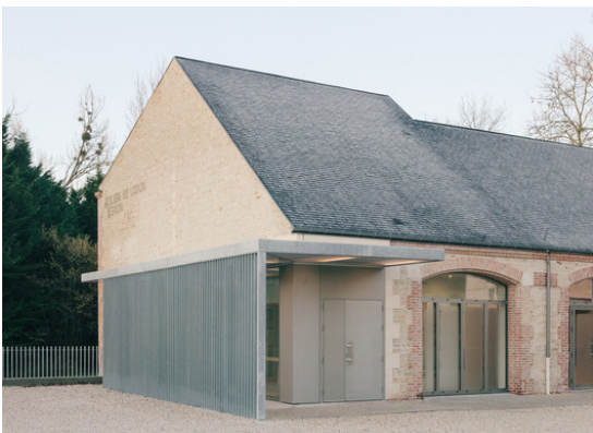
Single storey on south with double storey to the north
