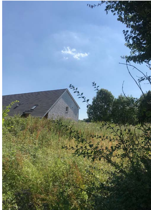
5 Low-Energy Affordable Homes, Chrishall, Cambridgeshire
