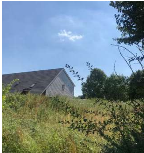
5 Low-Energy Affordable Homes, Chrishall, Cambridgeshire
